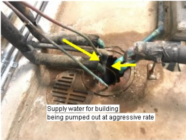
Water main is holding water and needs a sump pump
