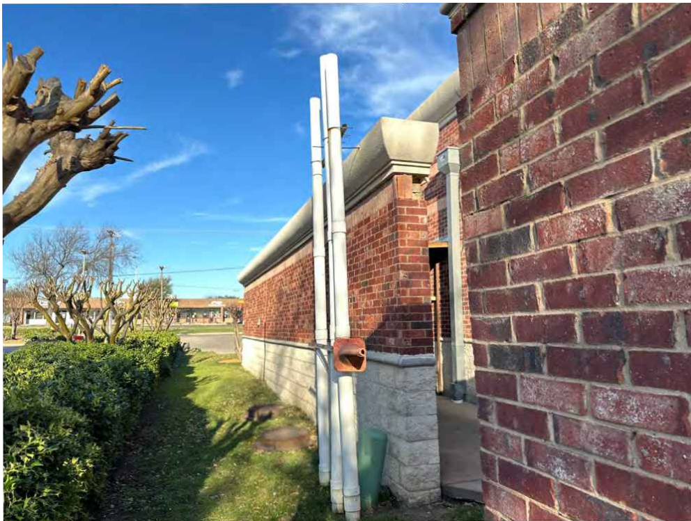
Photo 6 - View of the grease trap and plumbing vent pipes to the south of the building.
