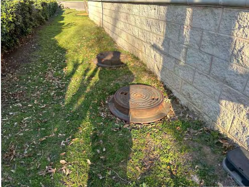
Photo 7 - Close-up view of the grease trap.
