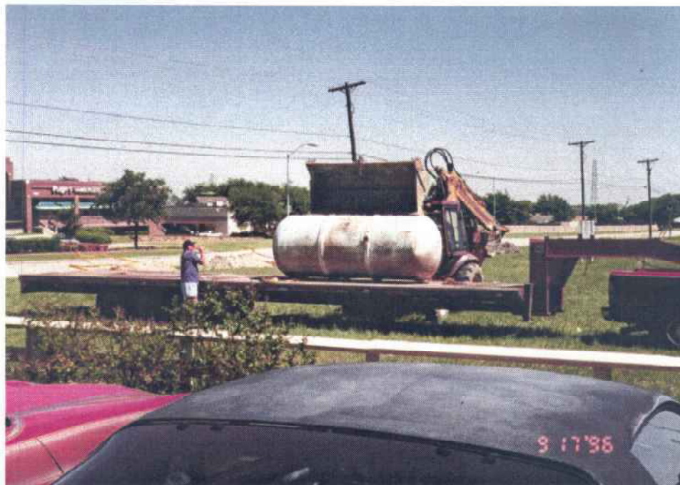
Photo 2: View of UST being loaded for transport to Hughes Tank Company of Venus, Texas, for disposal.
