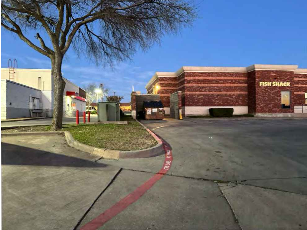
Photo 3 - View of the south side of the Subject Property, looking westward.
