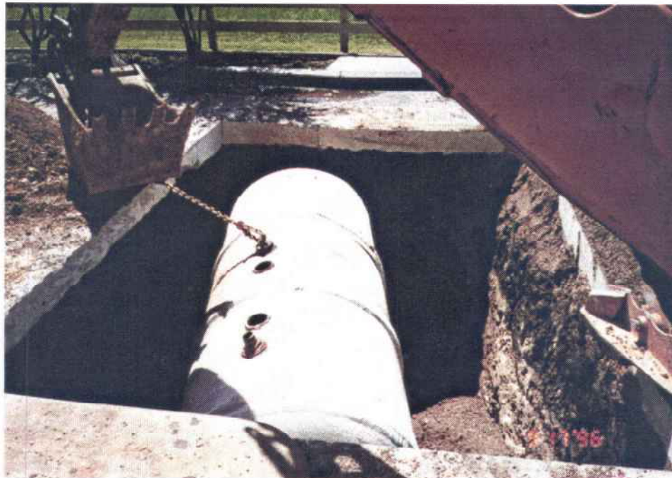
Photo 1: View of used oil UST before removal, Exxon 6-0426, 1400 E. Campbell Road, Richardson, Texas.
