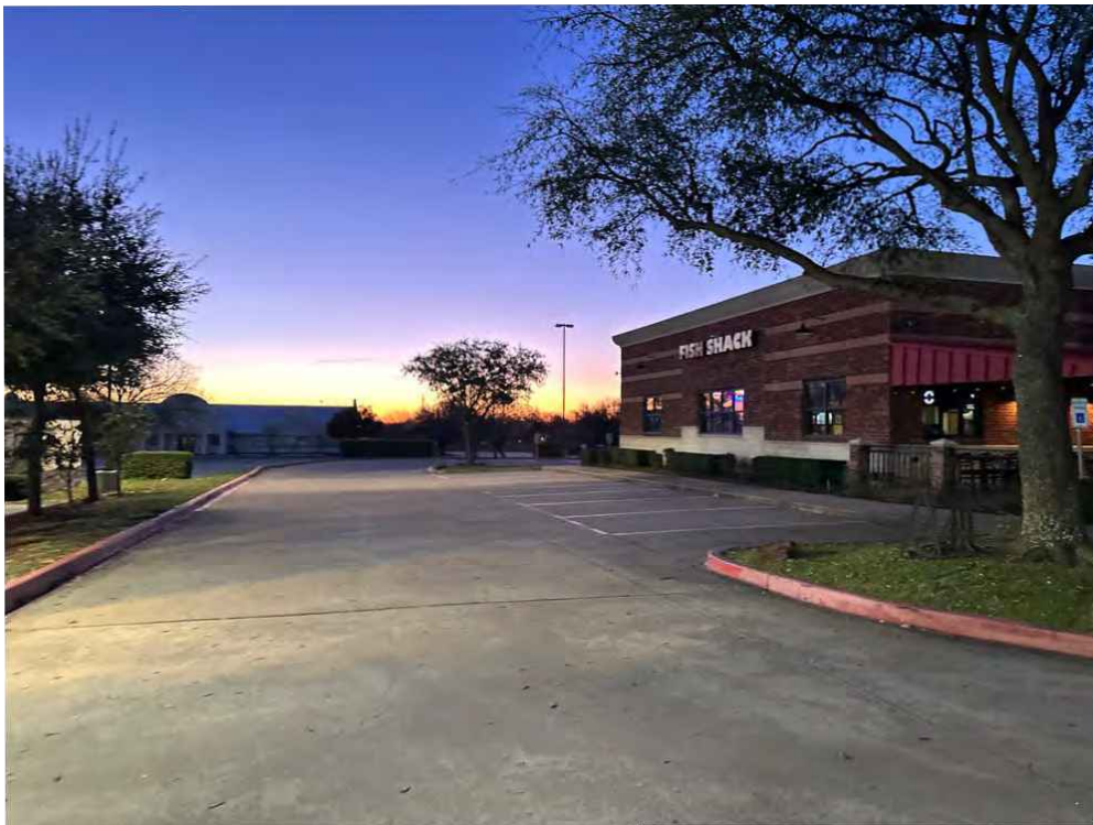
Photo 2 - View of the north side of the Subject Property, looking eastward.
